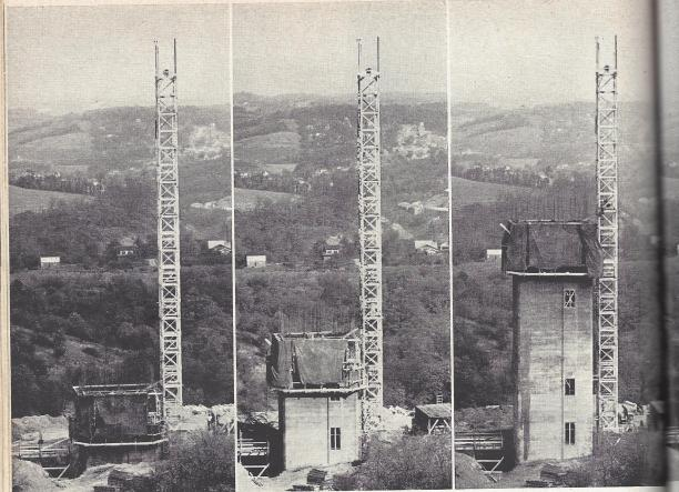
How a concrete building lifts itself by its own bootstraps is shown in the series of pictures above, made from the same location during the
